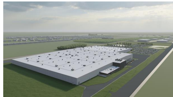
Magna Electric Vehicle Structures planned expansion in St. Clair
